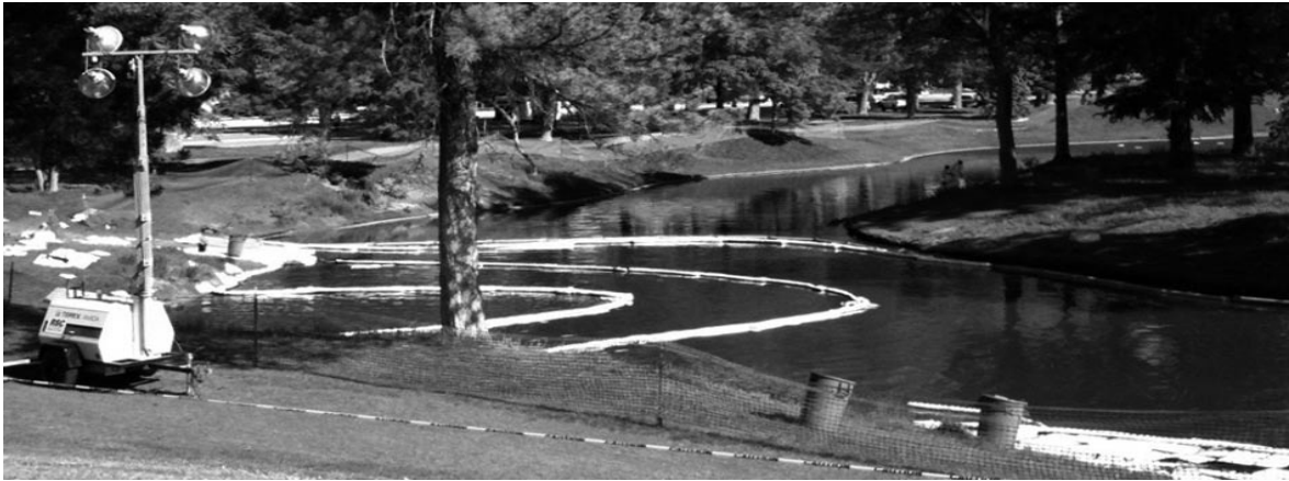
Oil-trapping booms appear in Liberty Park's lake to collect the stuff from the spill in Red Butte canyon.
